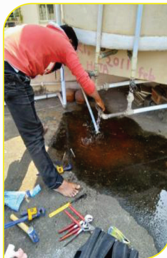
(Water tank Repairing Work)
