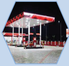
Essar Petrol Pump :- 200m
