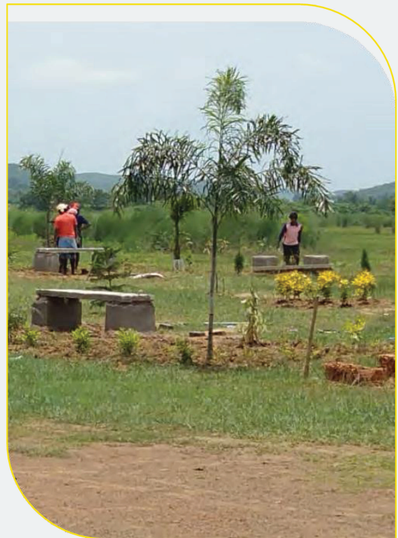
(Park work in progress)
